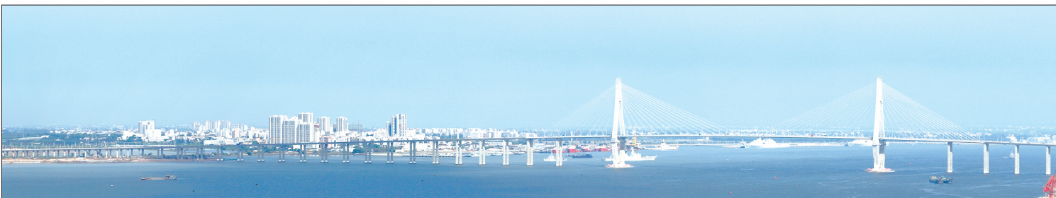
Zhanjiang Bay Bridge is among the longest cable-stayed bridges in the world.
